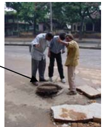
Excavation to verify the material used and measure the depth of the Manhole
